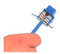
The keystone jack will then be placed in wall outlet and labeled with "D" for data. Example V1 would be voice 1 and connected into the proper switch and will correspond with the number on the patch panel. See below photo of example:
